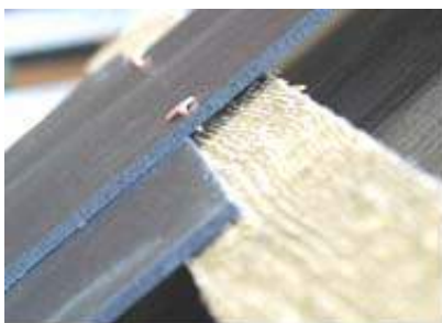
Slates fixed to 116mm headlap
