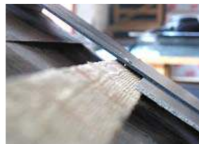
Slates fixed to 72mm headlap
